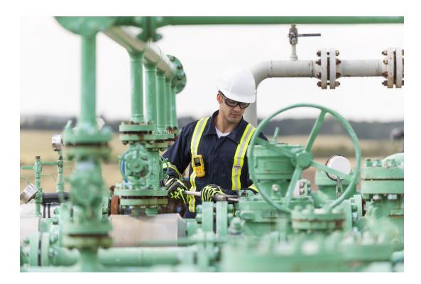
Measuring the lower explosive limits of combustible gases is essential in the construction industry. A gas leak can occur at any time, endangering the lives of workers and clients. If these gases reach a certain threshold, the gas could combust, leading to a flash fire or explosion. Construction managers and business leaders need to understand how LEL gas monitors function in the workplace to keep their workers safe.
